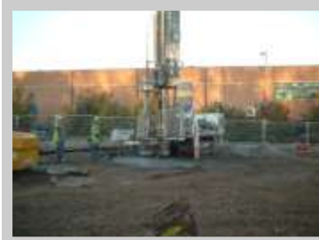
Ground Source Heat Pump Drilling Rig
