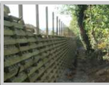
Cribblock Retaining Wall
